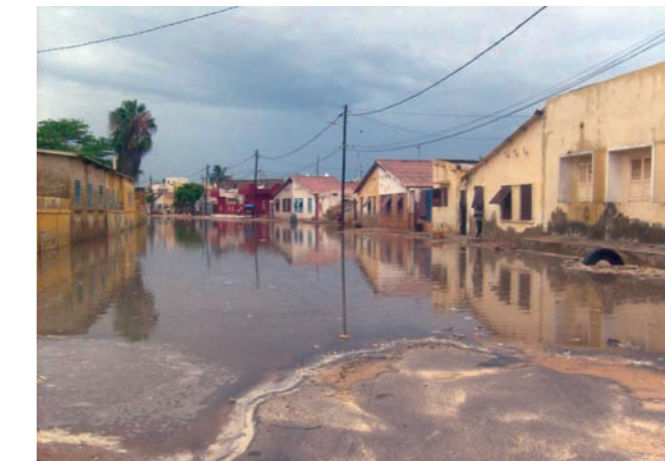
Flooding in Saint Louis.
