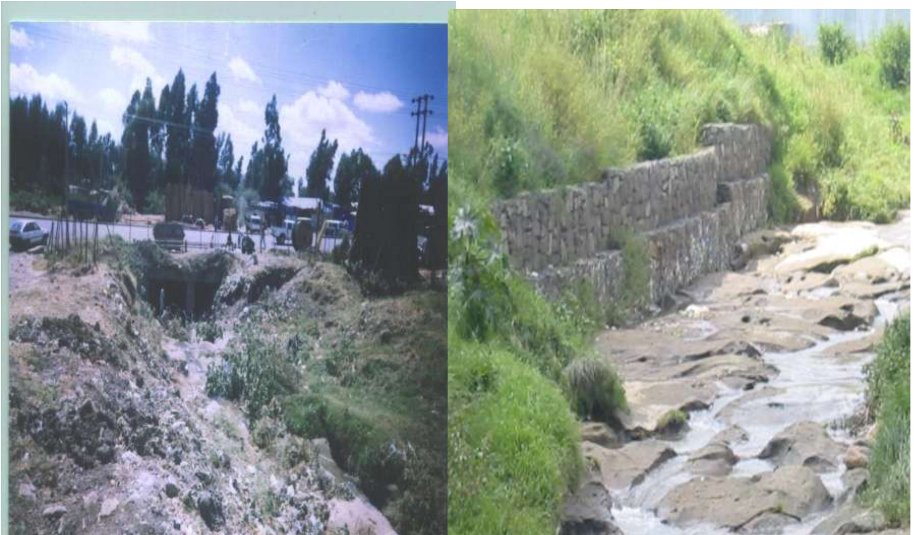
Jelisa river before and after rehabilitation
